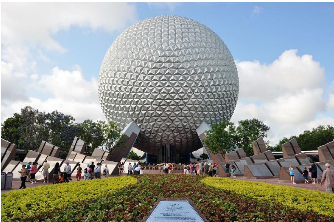
Figure 43: Spaceship Earth structure at Epcot Theme Park
